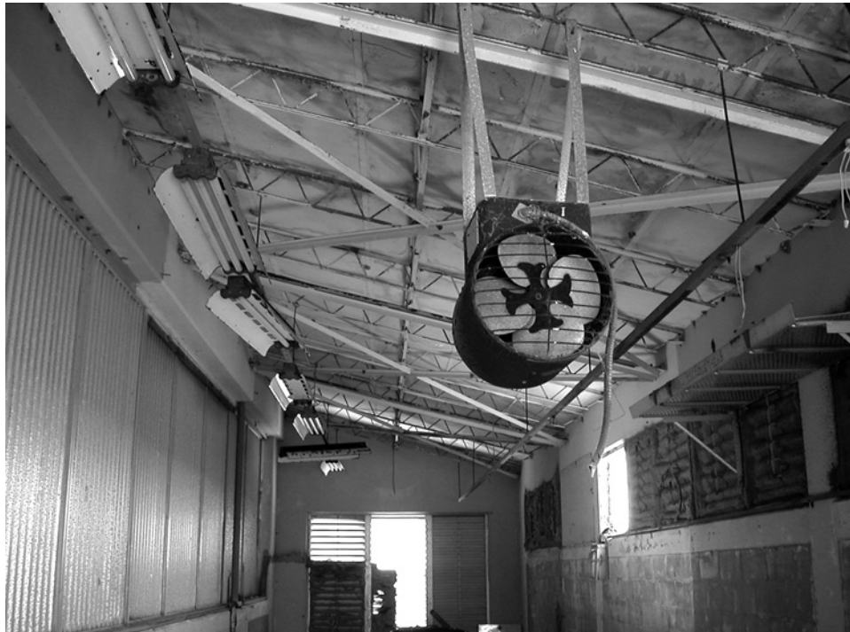
Figure 56. Interior of optical alignment building 32 showing roof joists and lighting (ERDC-CERL 2007).
