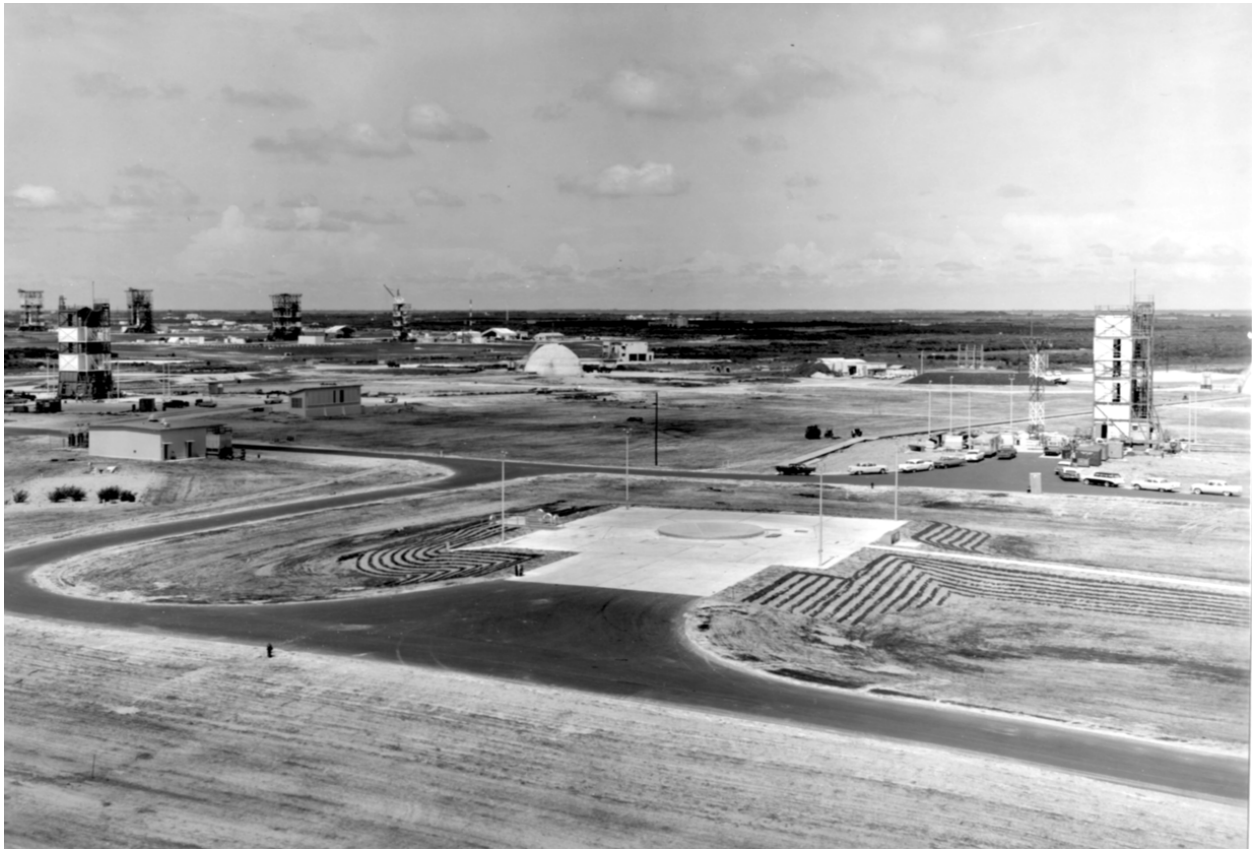
Figure 17. Completed silo 32B, 18 July 1960 (NARA).
