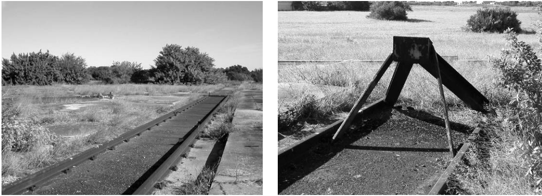
Figure 63. Pad 32 rail spur and bumper (ERDC-CERL 2007).
