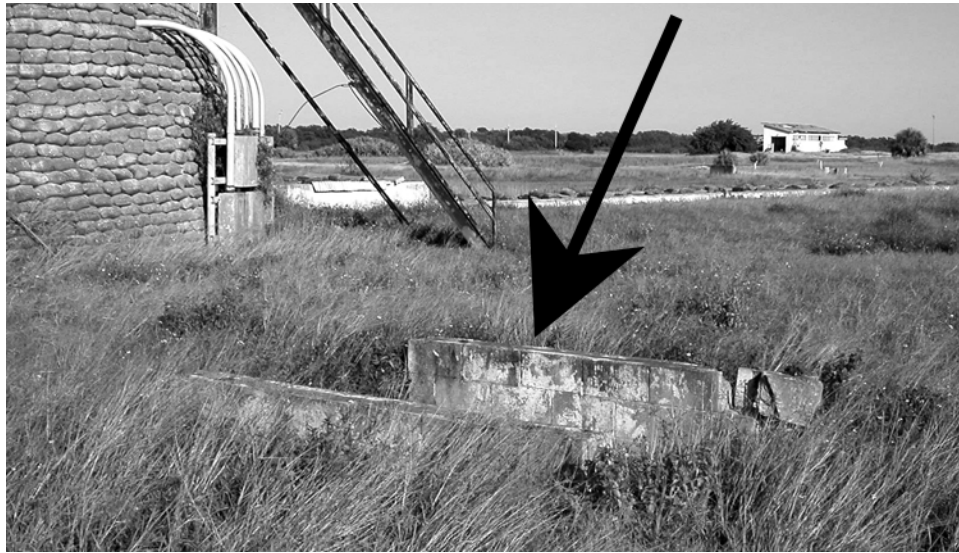
Figure 53. Blockhouse 31 cooling tower walls (ERDC-CERL 2007).
