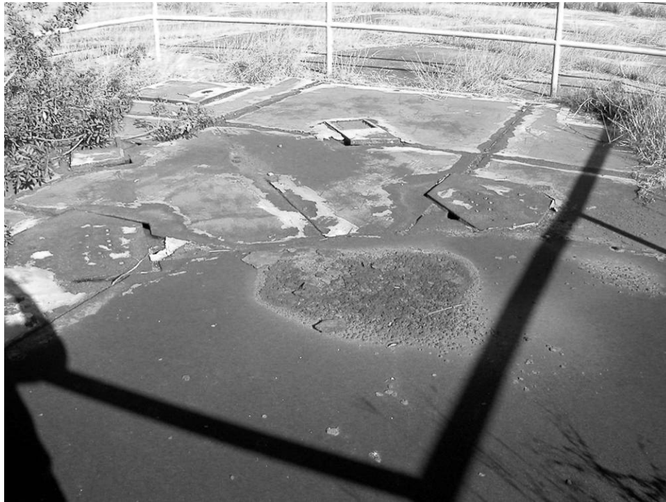
Figure 45. Pad 31 firing pit covered with metal plates (ERDC-CERL 2007).
