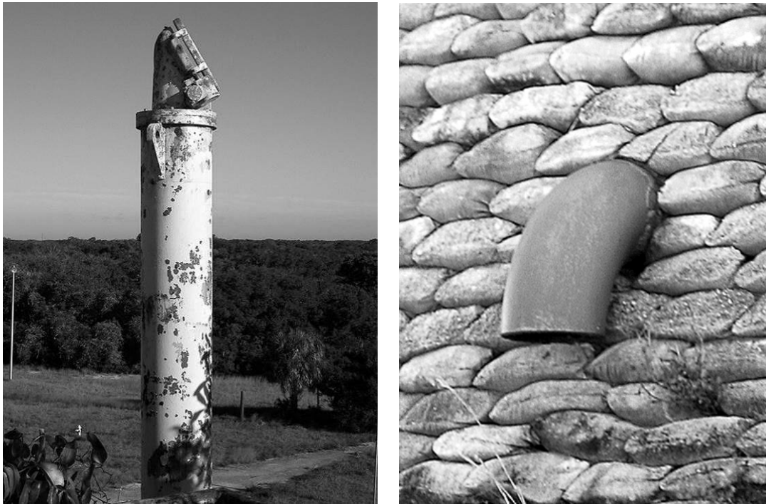
Figure 50. Blockhouse 32 periscope (left); toilet exhaust pipe (right) (ERDC-CERL 2007).
