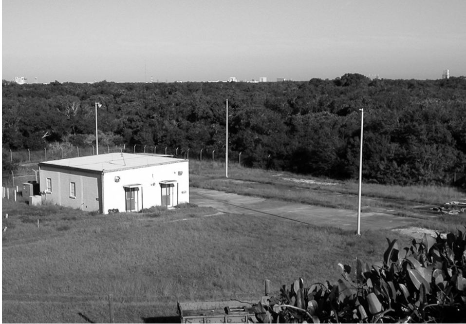
Figure 61. The MUSF support shop and its track bed (ERDC-CERL 2007).
