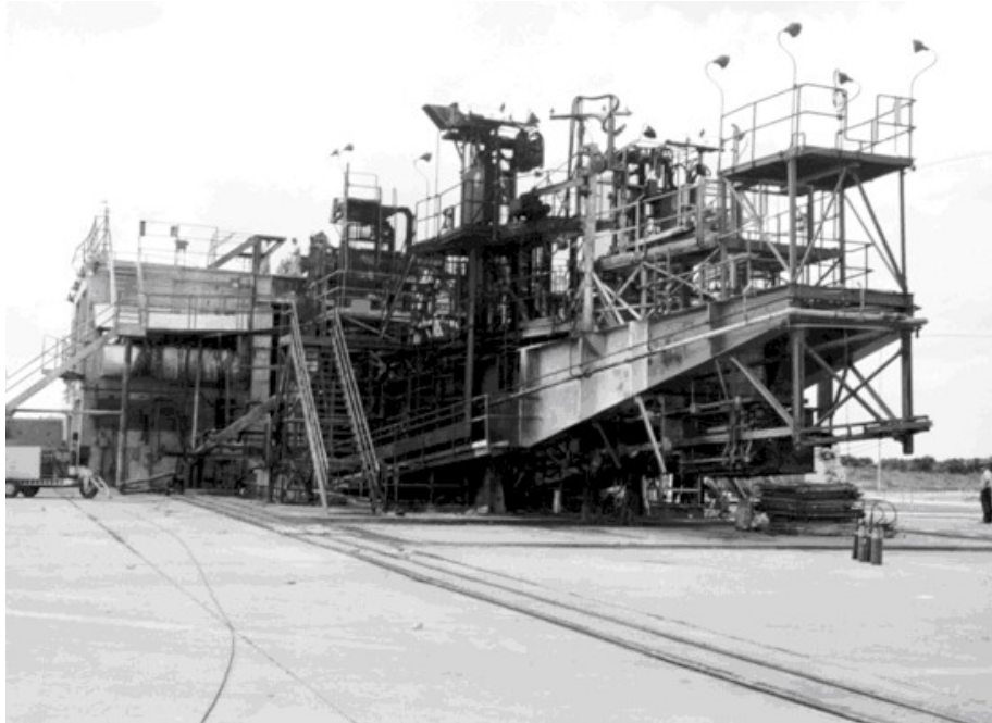
Figure 9. Navaho launch pedestal and gantry, 3 May 1957 (NARA).
