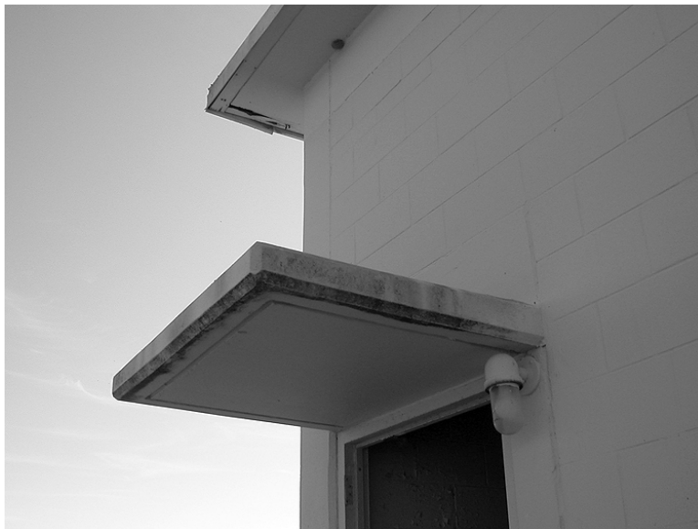
Figure 64. Launch support building eave and entry canopy (ERDC-CERL 2007).
