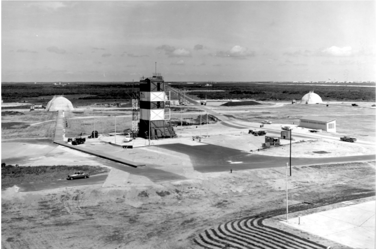
Figure 19. View of completed complex 31 with blockhouse to left, pad A in center, and silo B at near right, 18 July 1960 (NARA).
