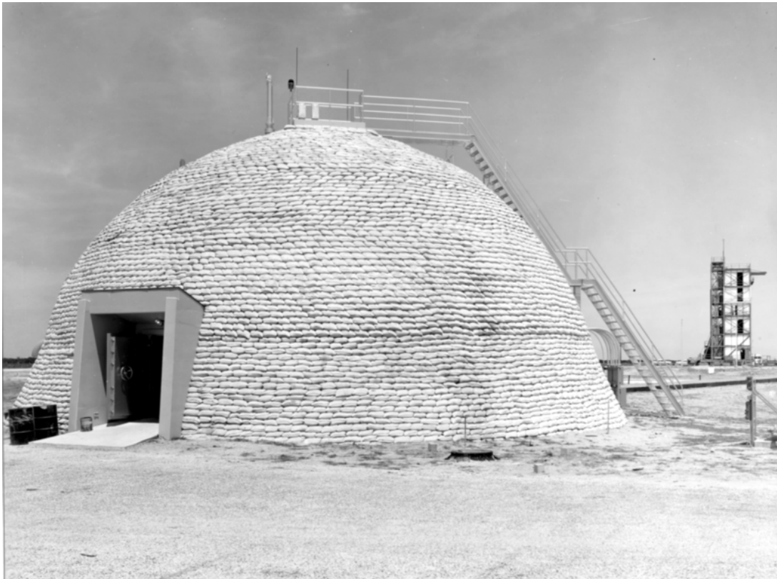
Figure 14. Completed Blockhouse, 18 July 1960 (NARA).
