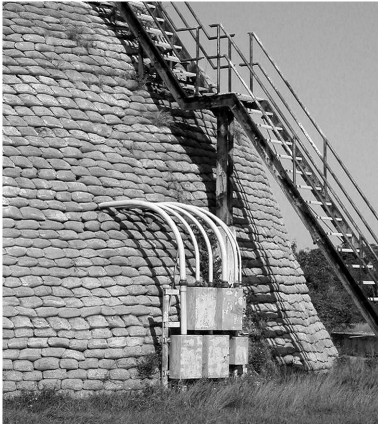
Figure 52. Blockhouse 32 electrical conduit sleeves and pull boxes (ERDC-CERL 2007).
