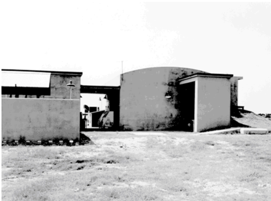
Figure 10. Blockhouse, transformer vault, and nitrogen shed at complex 9/10, 8 June 1956 (NARA).
