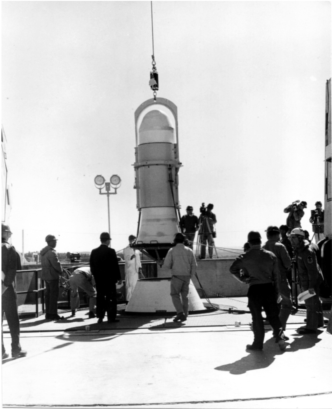
Figure 32. Nose cone being positioned on Minuteman I missile on launch pad, 1961 (NARA).
