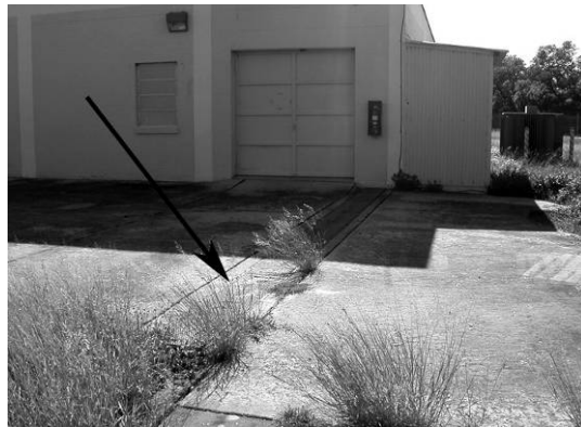
Figure 62. Riveted utility trench cover (left); north-south utility trench between MUSF support shop and track bed (right) (ERDC-CERL 2007).
