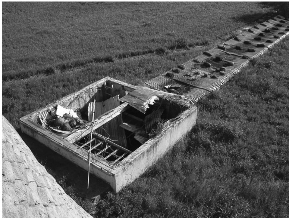
Figure 72. Cableway transition I behind blockhouse 32 (ERDC-CERL 2007).
