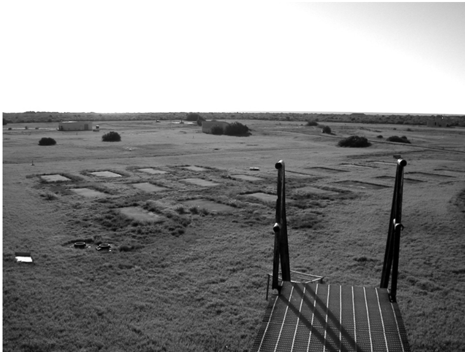
Figure 44. Tent pads constructed near Blockhouse 32 (ERDC-CERL 2007).
