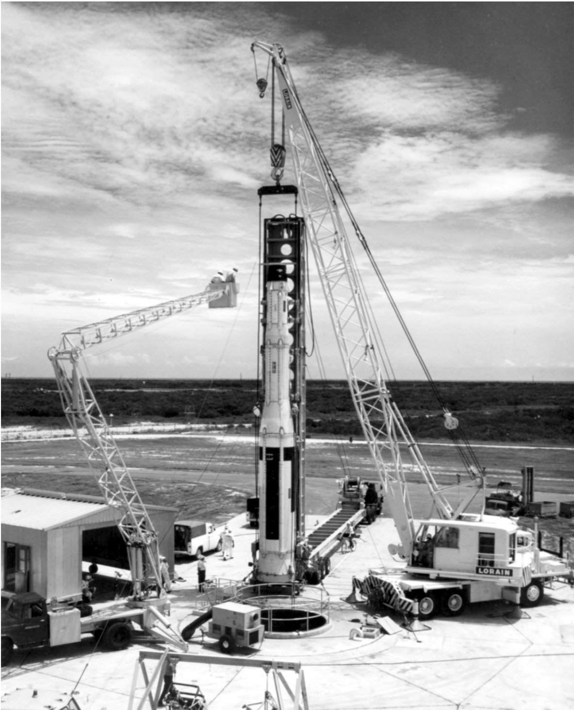
Figure 31. Minuteman I lifted from transporter/erector for lowering into silo (NARA).
