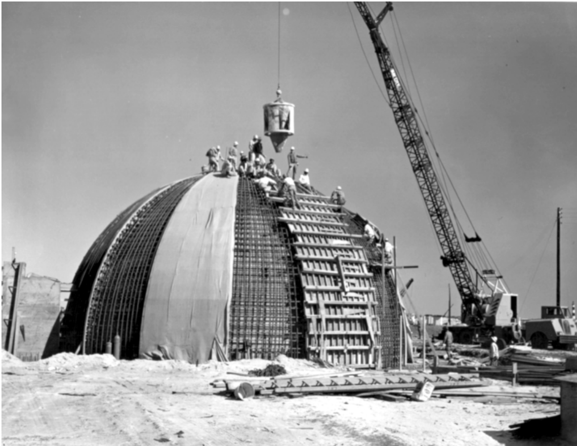
Figure 13. Pouring concrete for Blockhouse 31, 25 November 1959, (NARA).
