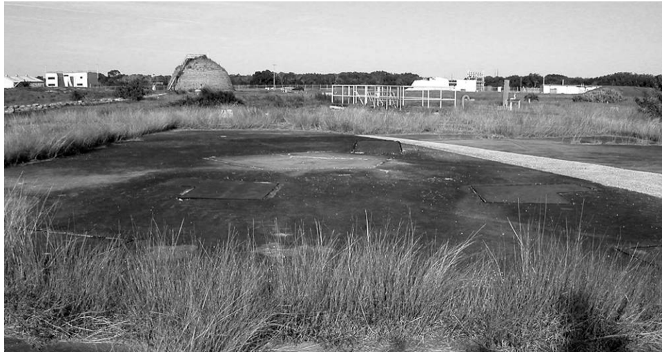
Figure 43. Navaho ramjet test pad at pad 31 (ERDC-CERL 2007).
