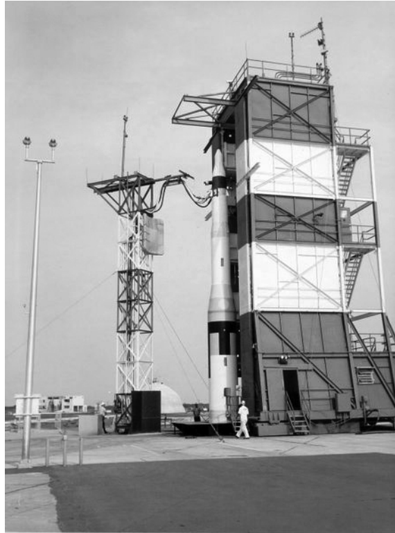
Figure 47. Pad 31 showing umbilical tower, launch stand, Minuteman I, and mobile service tower (PAFB n.d.).
