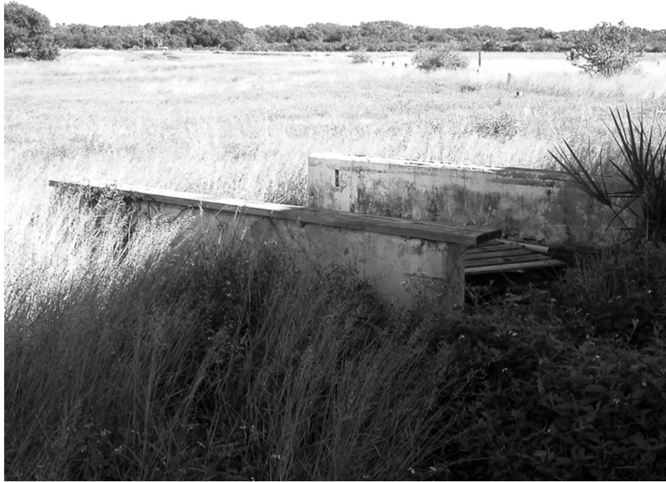
Figure 66. Launch support building cooling tower walls (ERDC-CERL 2007).
