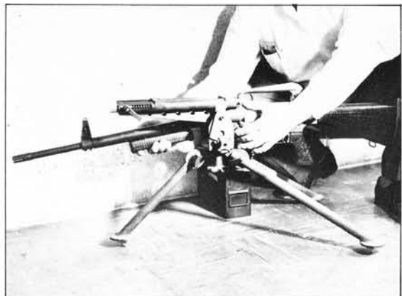
Barrel changing on the machine gun version of the AR-10 ( Armalyte Inc )
